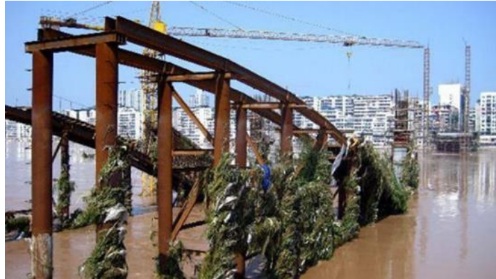
Figure 2. Collapse of Second Qujiang Bridge.
