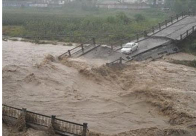
Figure 6. Collapse of Chongzhou Huaiyuan Bridge.
