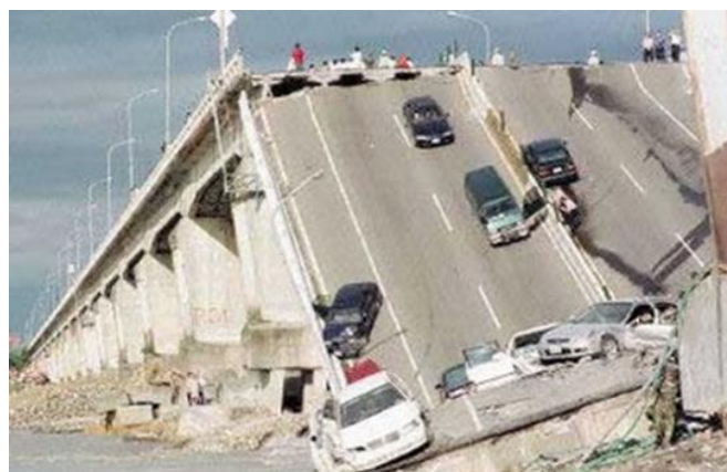
Figure 1. Collapse of Gaoping Bridge.
