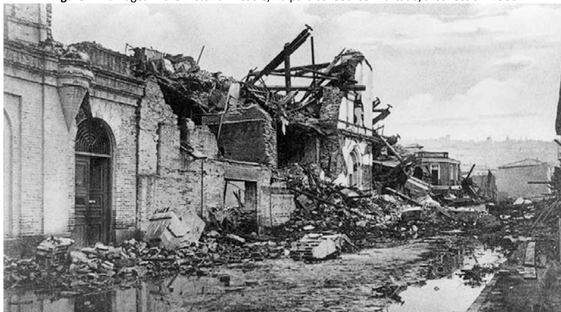
Figure 1. Damages in the Victoria Theatre, Valparaíso. Source: Hurtado, J. collection. 1906.
